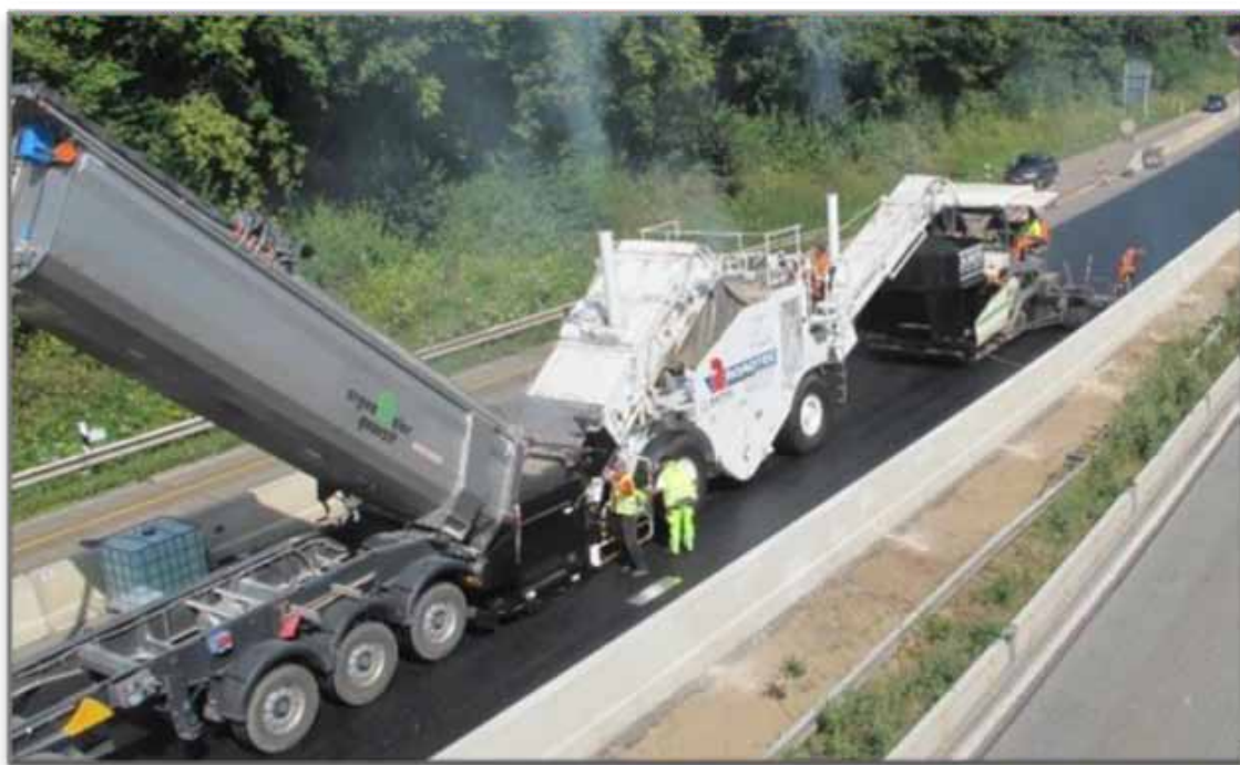
26. ábra: A Shuttle Buggy adagoló (ASTEC MOBILE MACHINERY GmbH, 2019).
